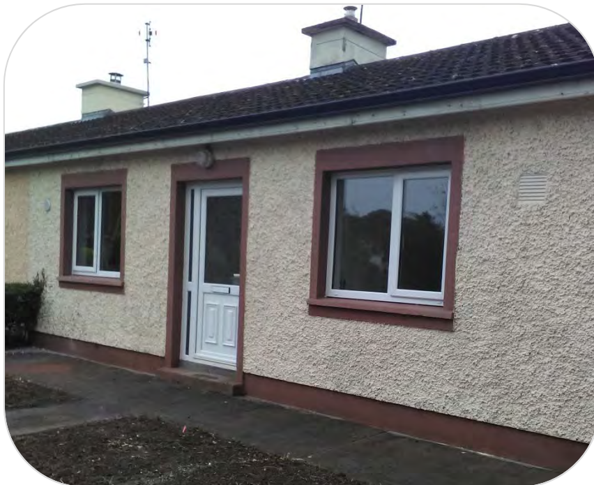
Housing Maintenance project at 64 Shannon Park Portumna
