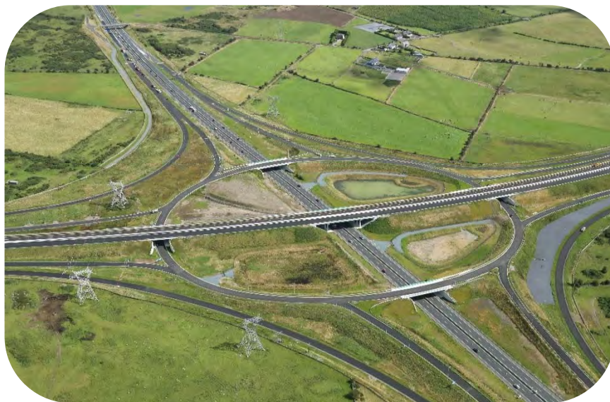
M17/M18 Rathmorrissey Junction
