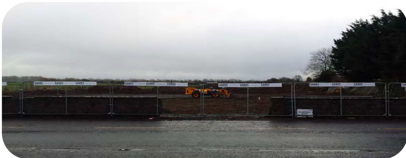
Tuam Fire Station new site December 2017
