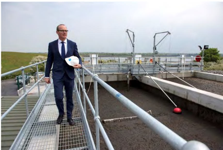
Minister Coveney at the official opening of Kinvara waste water treatment plant
