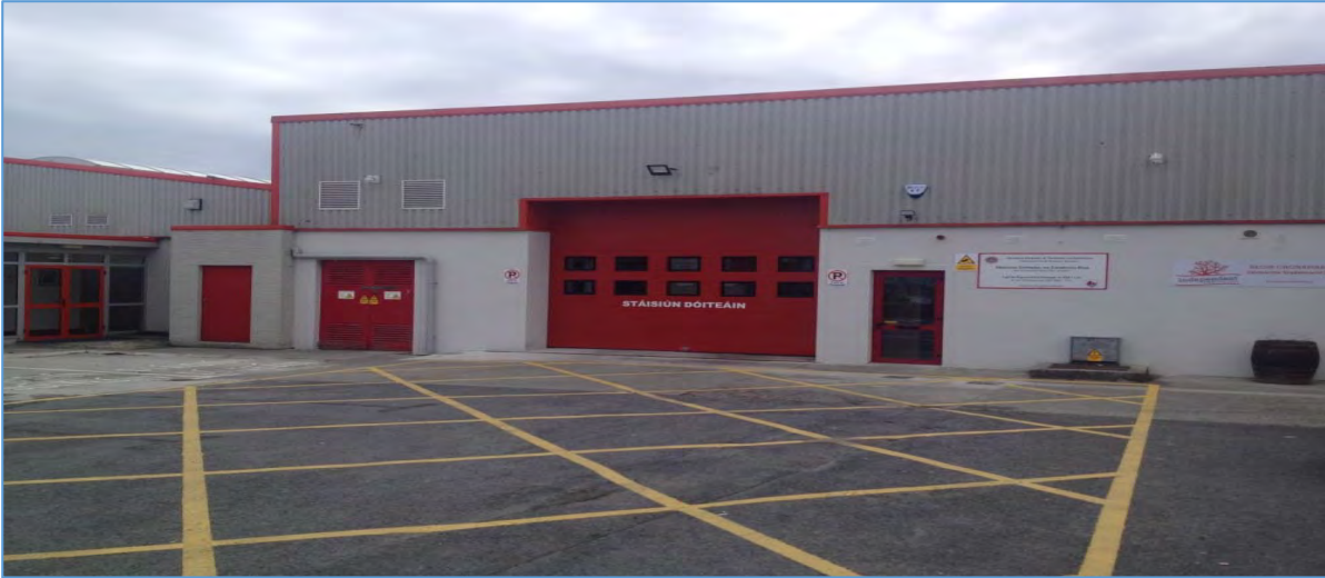
New Fire Station An Cheathrú Rua
