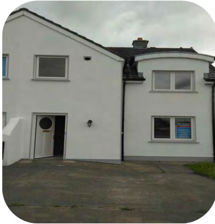
Housing Maintenance project at Weir Rd, The Pottery, Tuam.
