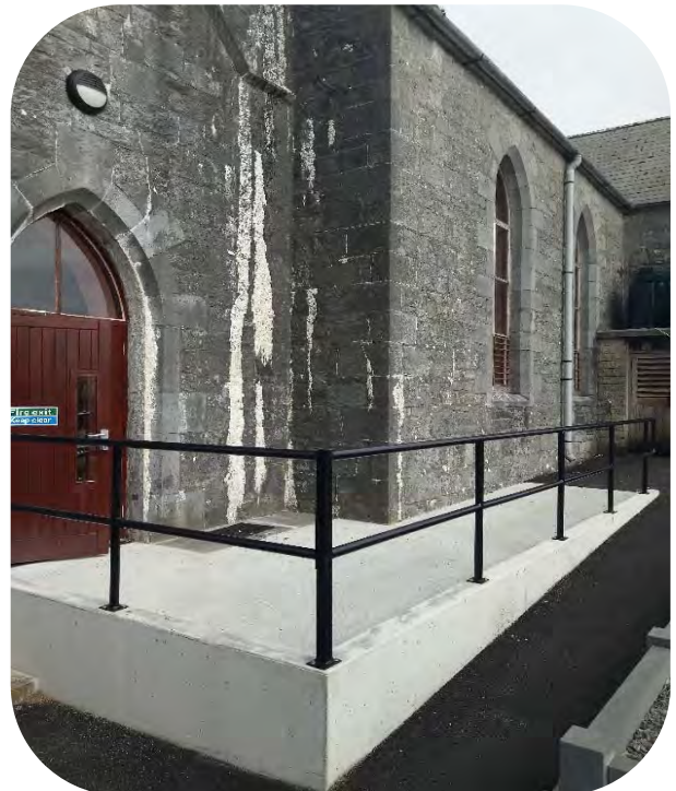
Accessibility works at Gort Library
