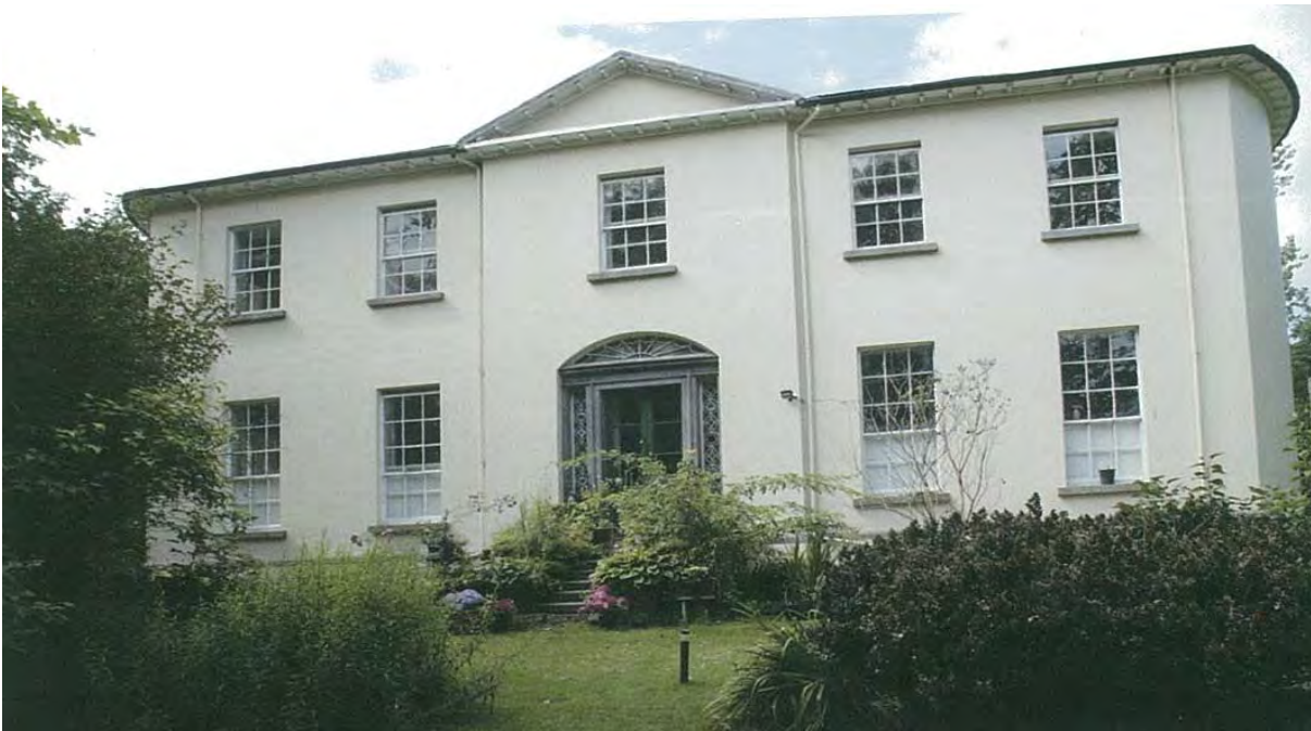
Roof repairs were carried out to Ballynagar House under the Historic Houses initiative of the Department of Culture, Heritage and the Gaeltacht
