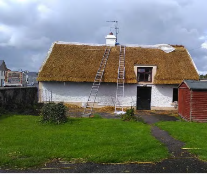
Thatch repair to house at Tynagh
